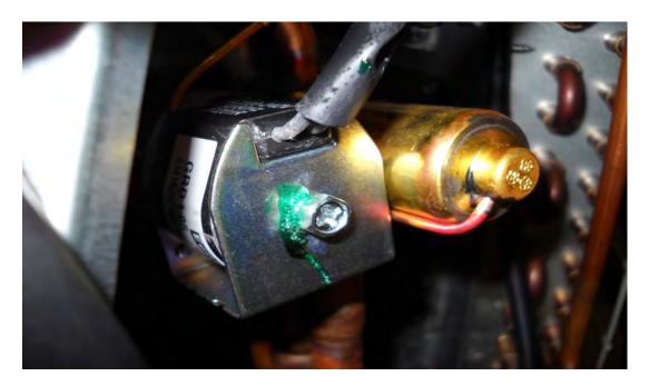
There's one reversing valve located below the control board assembly. The coil is replaceable, and can be checked out from the plug at the board.
