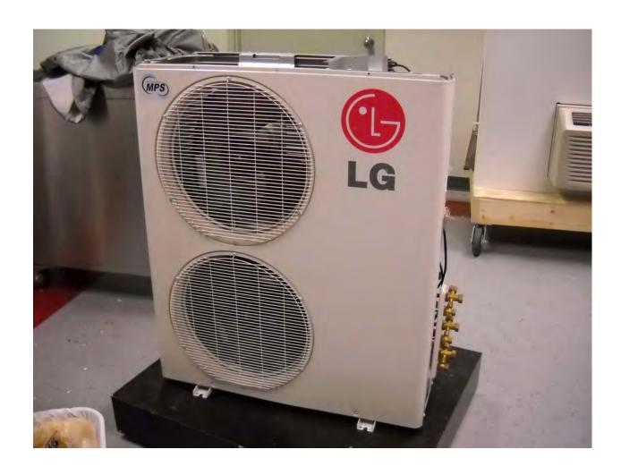
The machine pictured here is setup for up to three indoor units. This is shown by the three sets of brass fittings for the refrigerant lines on the side of the machine.
