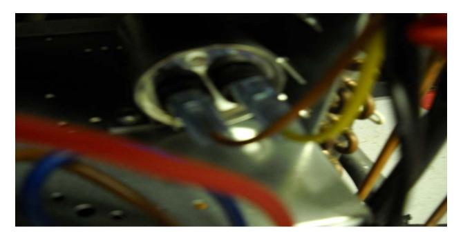
The capacitor for the outdoor fan motor is located below the control board assembly. This is one of the reasons it is advantageous to check components out at the plug rather than having to dig down to where they're located.
