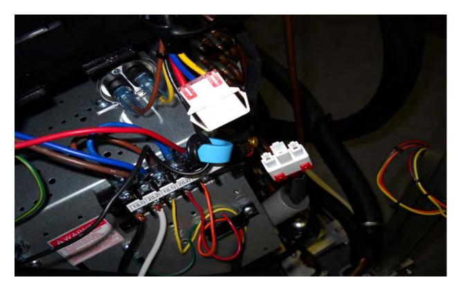
With a plug open on the plug side going to the compressor we can check the windings of the compressor. We can check winding to winding and winding to ground. Since this is a three phase compressor, there is no capacitor. If we were working on a standard compressor we would be able to shut off the power and read the capacitor at the receptacle side of this plug.
