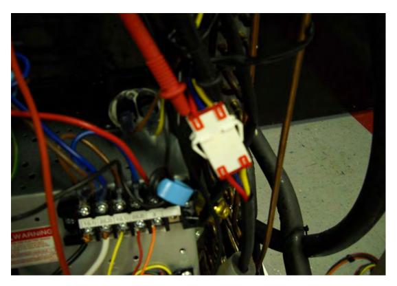
At the three wire compressor plug we can check voltage to each lead and the frequency going to the compressor.
