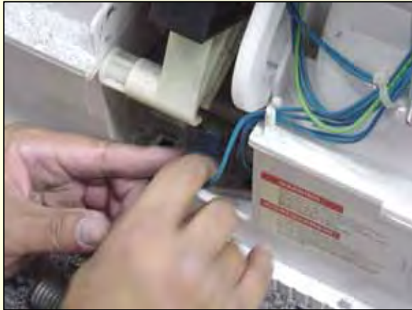
Disconnect drain pump wires
