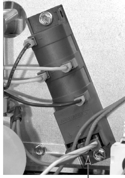
2 Wht/Blu Ignition Switch Wires On Spark Module Terminals
