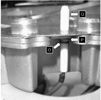
Crown burner orifice replacement
