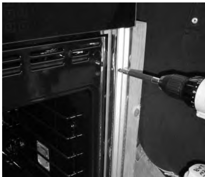
Oven Mounting Screw Locations
