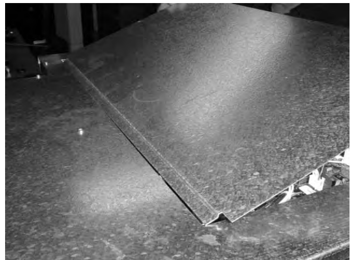
Replacing the Access Panel
