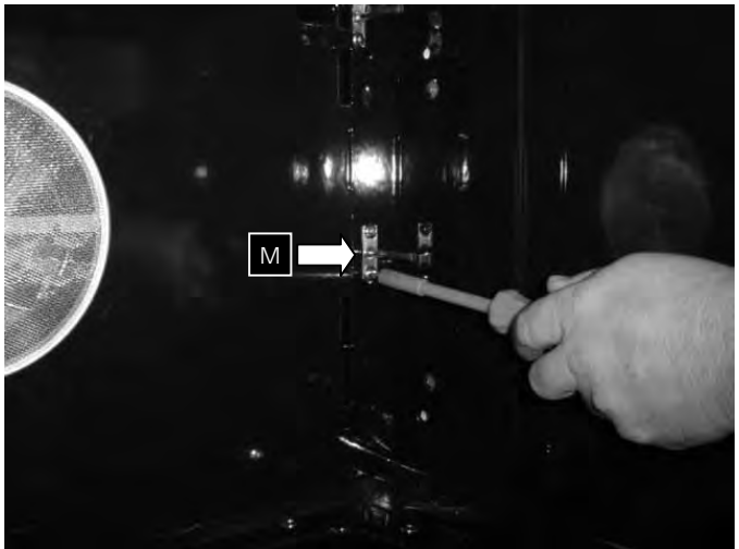
Temperature Sensor (1 of 3 Inside Oven)
