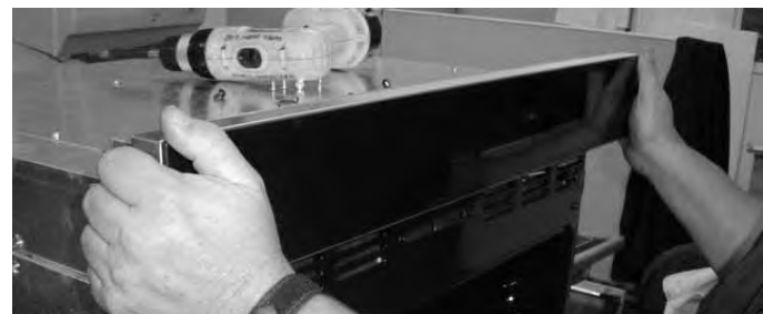
Control Panel Removal
