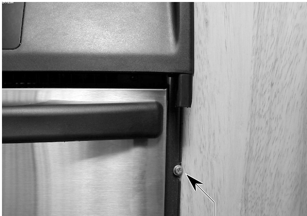
Cabinet Mounting Screw (2 Screws On Each Side)
