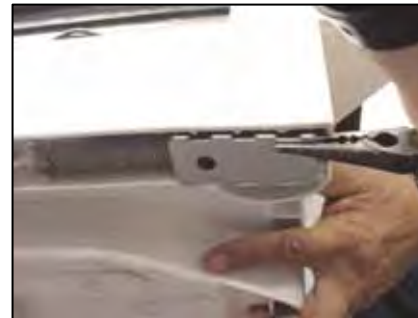
Pulling out door springs from base & disconnecting cords
