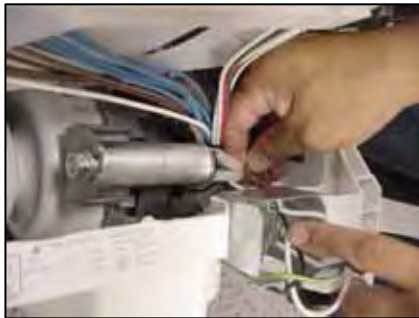
Pulling J-box wires
